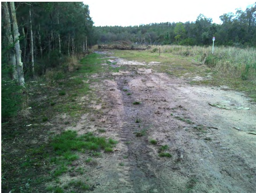
Plate 8 Cleared gas pipeline corridor, south eastern portion Lot 7.
