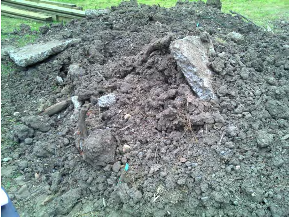
Plate 3 Demolition works, Lot 7.
